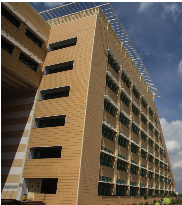
India's first commercial radiant cooled building, Infosys Software Development Building, Hyderabad, Andhra Pradesh, India.
