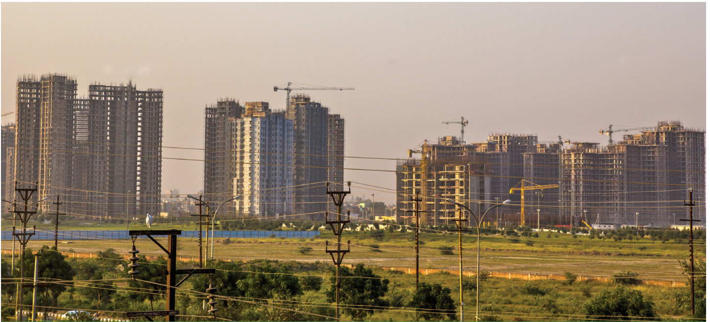
Construction underway in Greater Noida, Uttar Pradesh, India.
