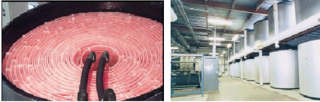
Fig. 4.2: Modern Ice Storage tanks with Brine filled Plastic tubes
